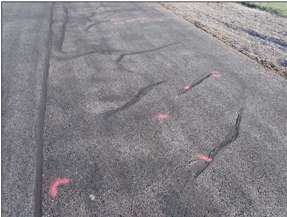
TW-11-02: L&T Cracking
