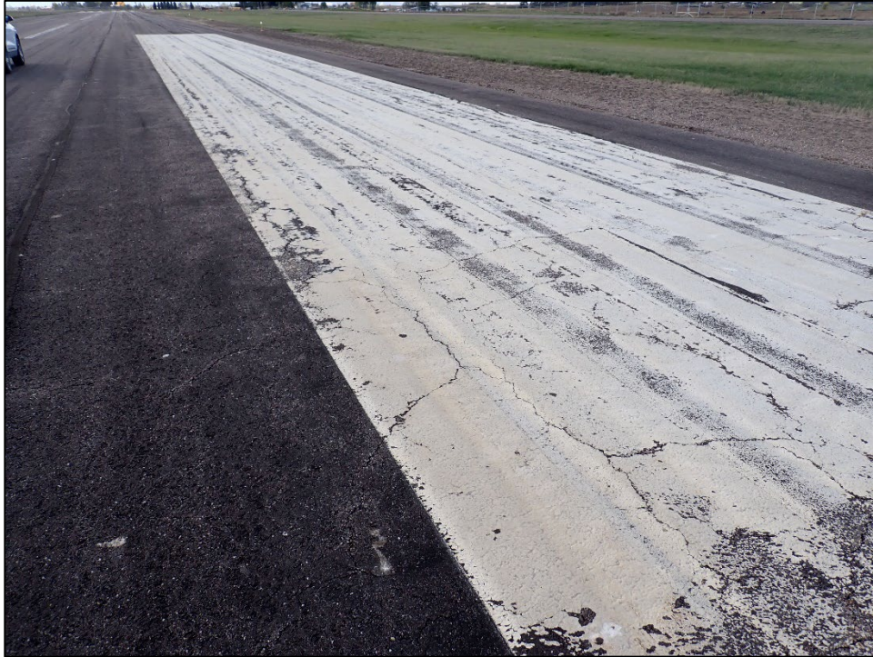
RW16-11-18: L&T Cracking
