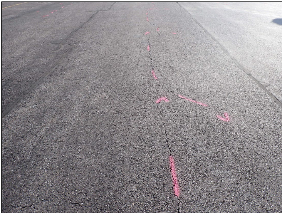
AP-11-21: L&T Cracking
